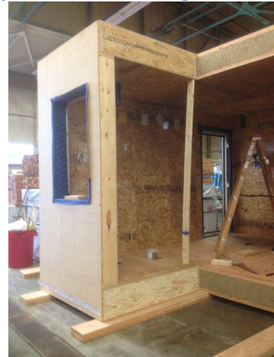
Figure 2 Assembly of House for Testing
