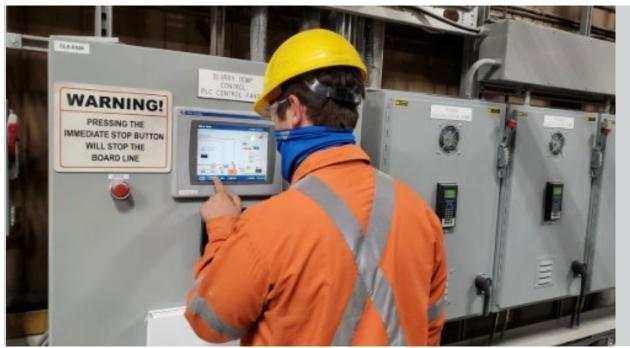
Process Engineer Loren Olshansky, works at the Slurry Temperature Control panel to monitor the boiler temperature setting.
