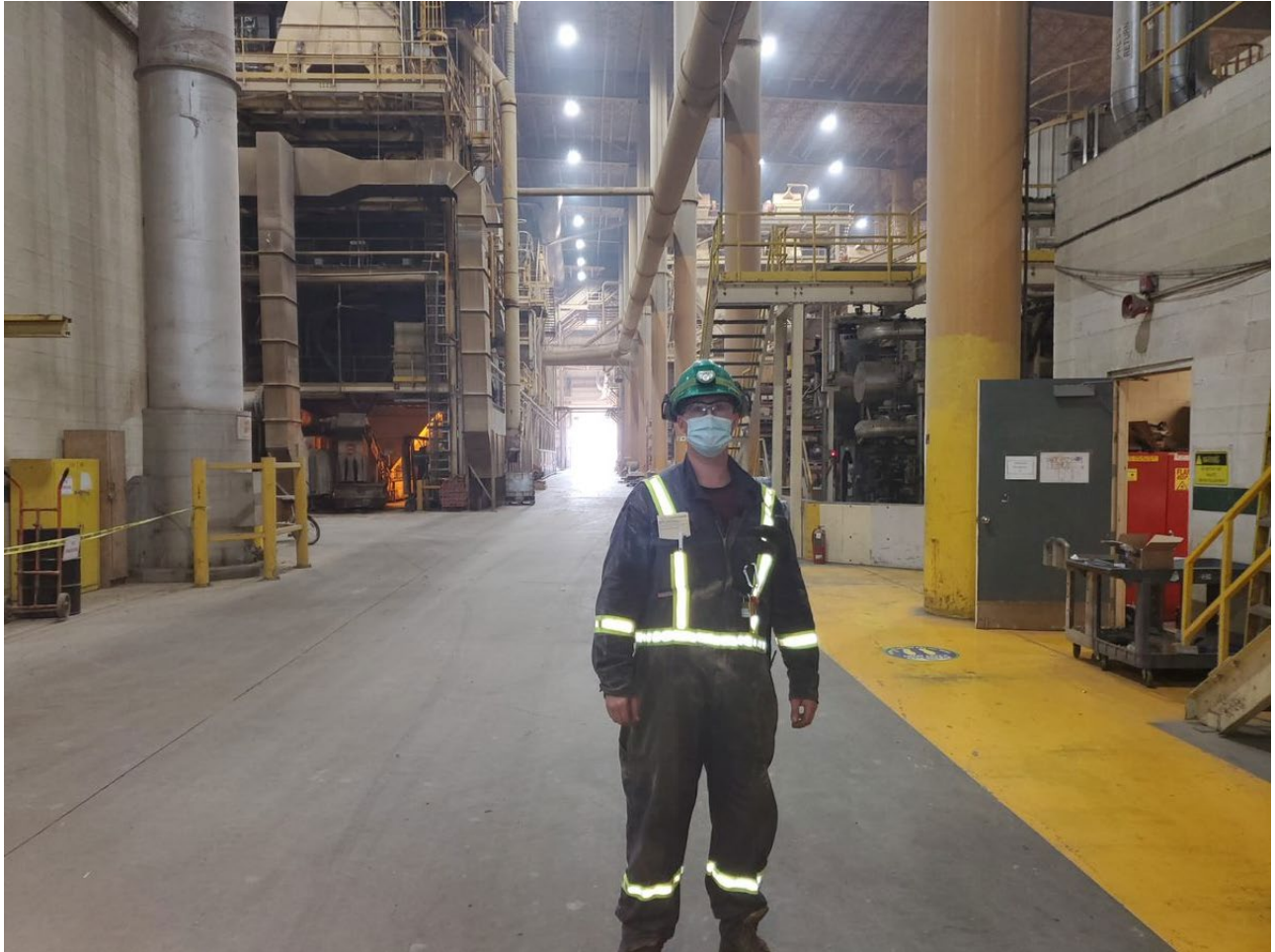
Joe Barth stands beneath the new and more energy efficient LED high bay lights.
