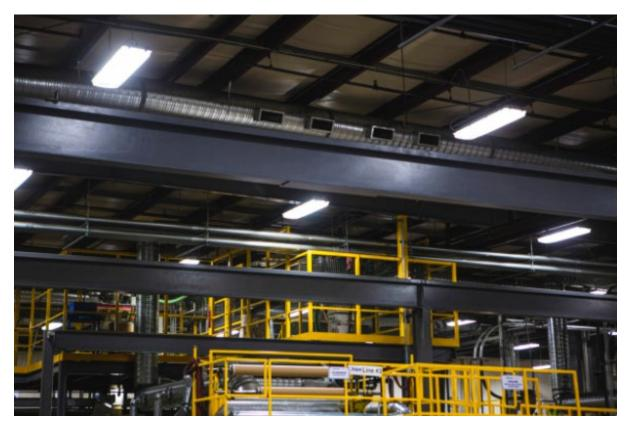
The completed LED lighting conversion across Orion's manufacturing plant provides brighter light while reducing electricity use.
