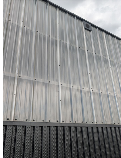
Left: The plant's south-facing wall, with the SolarWall system spanning the full height of the building. Right: close-up of the two-stage collector and outer glazing layer.
